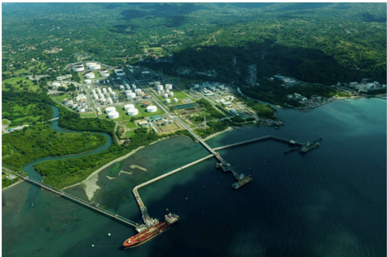
The Shell Tabangao refinery that will be converted into world-class import terminal
